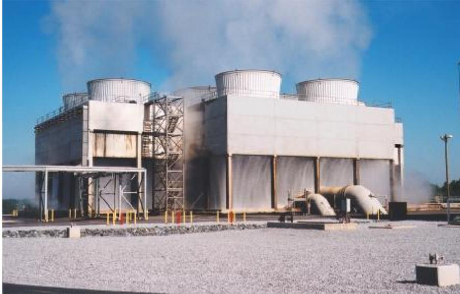
Open system cooling towers remove waste heat from the vapor cycle by exposing the cooling water directly to the atmosphere. After evaporation removes the heat, the remaining cooling water flows into the catch pool. Level control applications include a high level switch to avoid overflow from the cooling tower pool. In DC cooling systems, the inlet structure is usually a vertical sewage well pump, which requires high and low water level detection and possible pump control.
